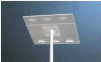
Wind channel structural back module support protects junction box and cabling
